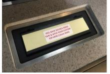
After ensuring that the Top is clean, dry and free from dust, peel back the tape and place the custom top into position. Press it firmly home. Allow 12hrs for adhesive to bond and cure.
