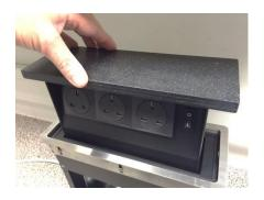
You can now add the required amount of extra weight into the recess, until you are happy with its pace of lift (when the new top is added more permanently later)
