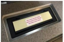
After ensuring that the Top is clean, dry <u>and free from dust</u>, peel back the tape and place the custom top into position. Press it firmly home. Allow 12hrs for adhesive to bond and cure.
