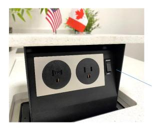
"If the receptacle senses any sort of an electrical overload or imbalance, it is designed to trip the circuit in a fraction of a second.
