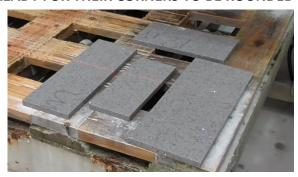
THE CORNERS ARE TYPICALLY ROUNDED BY HAND TO ENSURE THAT THE CUSTOM TOPS WILL NEATLY MARRY WITH THE INTERNAL RADIUS OF THE HOLES. THE EXPERIENCE AND SKILL OF THE WORKTOP SUPPLIER ENSURES THAT EVERYTHING WILL FIT BEAUTIFULLY ON SITE.
